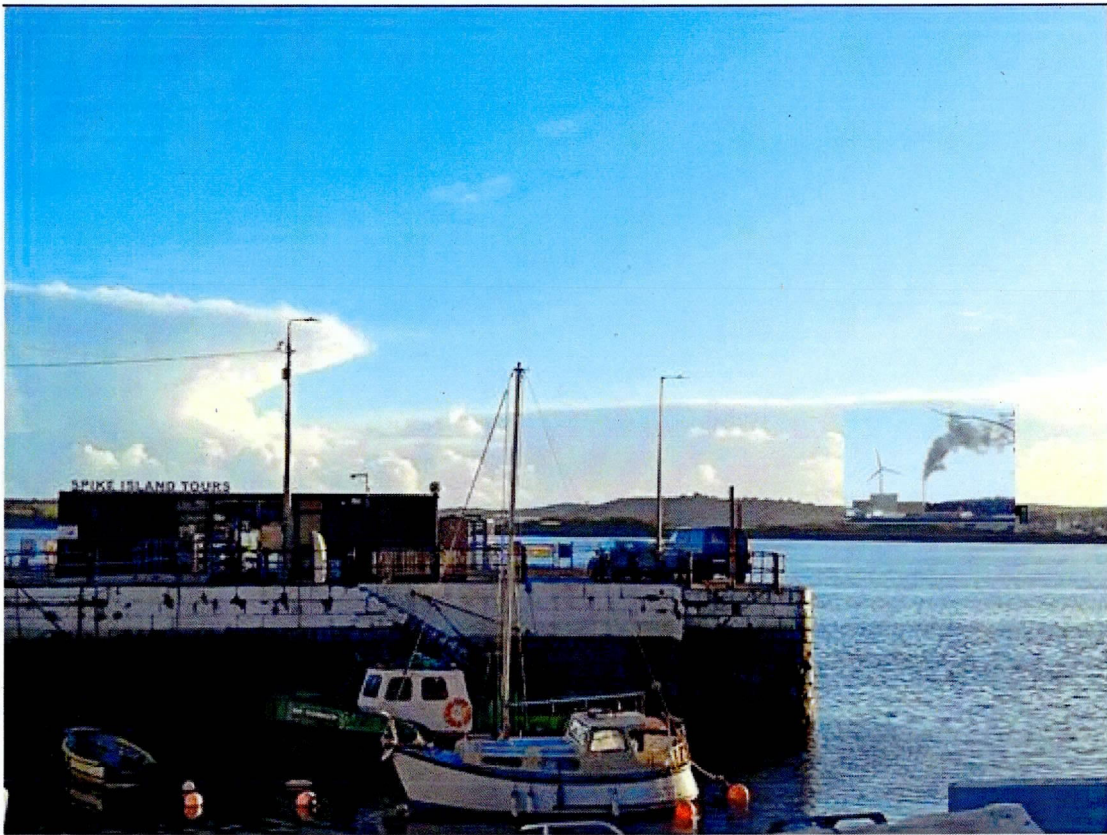
Plate 1: Potential view SSE from West Beach (town centre) to Spike Island ticket office and ferry departure point on Kennedy Pier.
